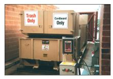
Also available with an advanced system for measuring and reporting container usage and fullness. Users can input an I.D. number to access the compactor.
